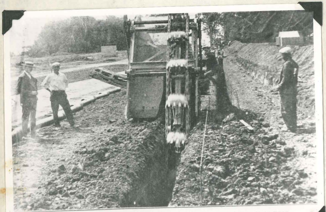
SERVICE AND WATER MAIN DUAL TRENCHING, MAIN STREET, FORT ERIE
